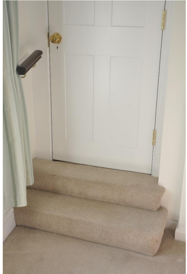
Photo 7 showing the steps (with handrail) from the Garden Suite to the main upstairs landing area.
